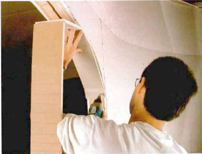
Like a rolltop desk. Scoring the backside gives \frac{1}{2} -in. drywall the flexibility to follow a curve. Screws must be placed carefully to avoid tearout.
