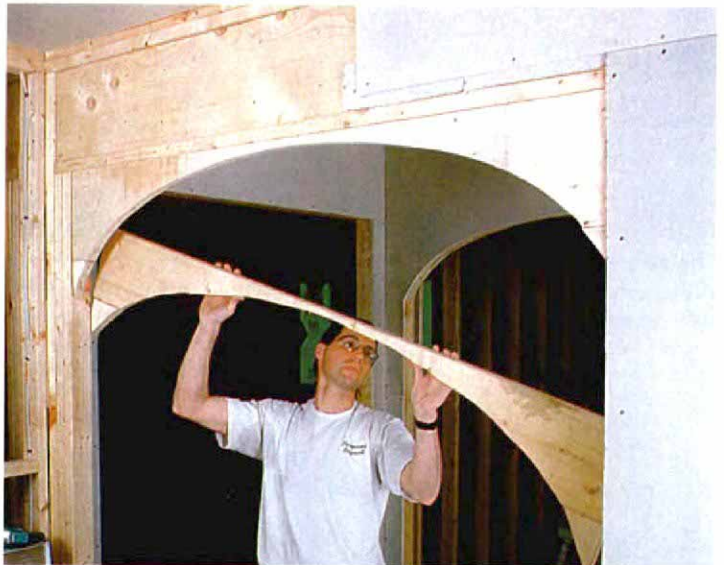
Framing is built up from dimensional lumber.
