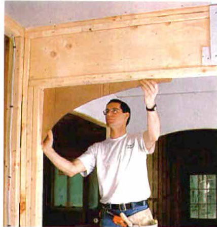
Layout begins with a cardboard template.
